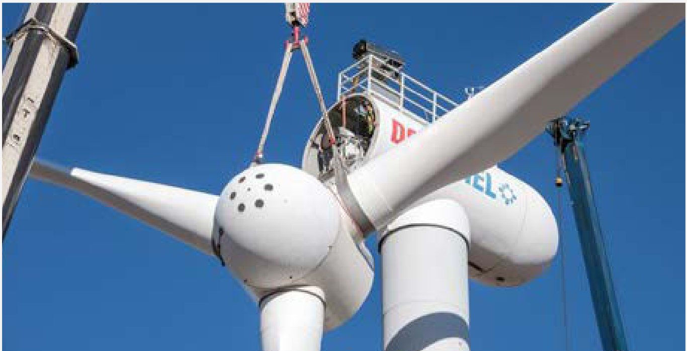
Scott Wilde, NREL research operations manager, peeks out of the nacelle of the three-bladed Controls Advanced Research Turbine (CART3) as he directs the two-crane operation to remove the turbine's rotor. Rotor blades specially designed by a research partner were then installed on the CART3 for a field validation campaign to take place during the windy winter season. Photo by Lee Jay Fingersh, NREL
