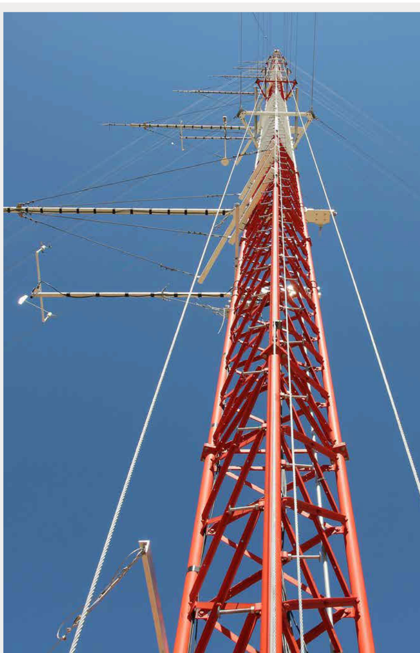
The U.S. Army utilized NREL's 135-meter meteorological tower to install instruments and collect data during a recent noise propagation experiment. Photo by Lee Jay Fingersh, NREL 40950
