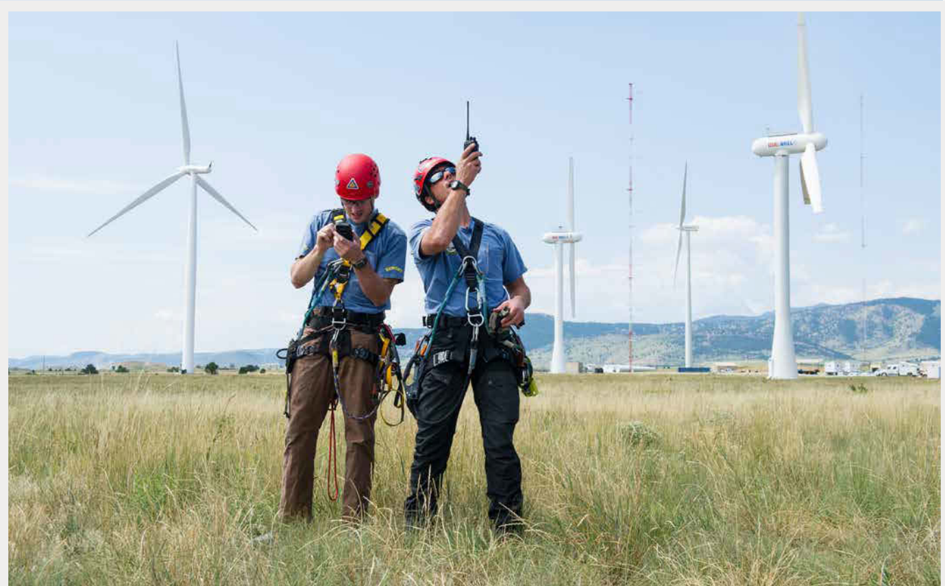
NREL researchers check the weather forecast and review safety plans before inspecting wind turbine blades. Photo by Dennis Schroeder, NREL
