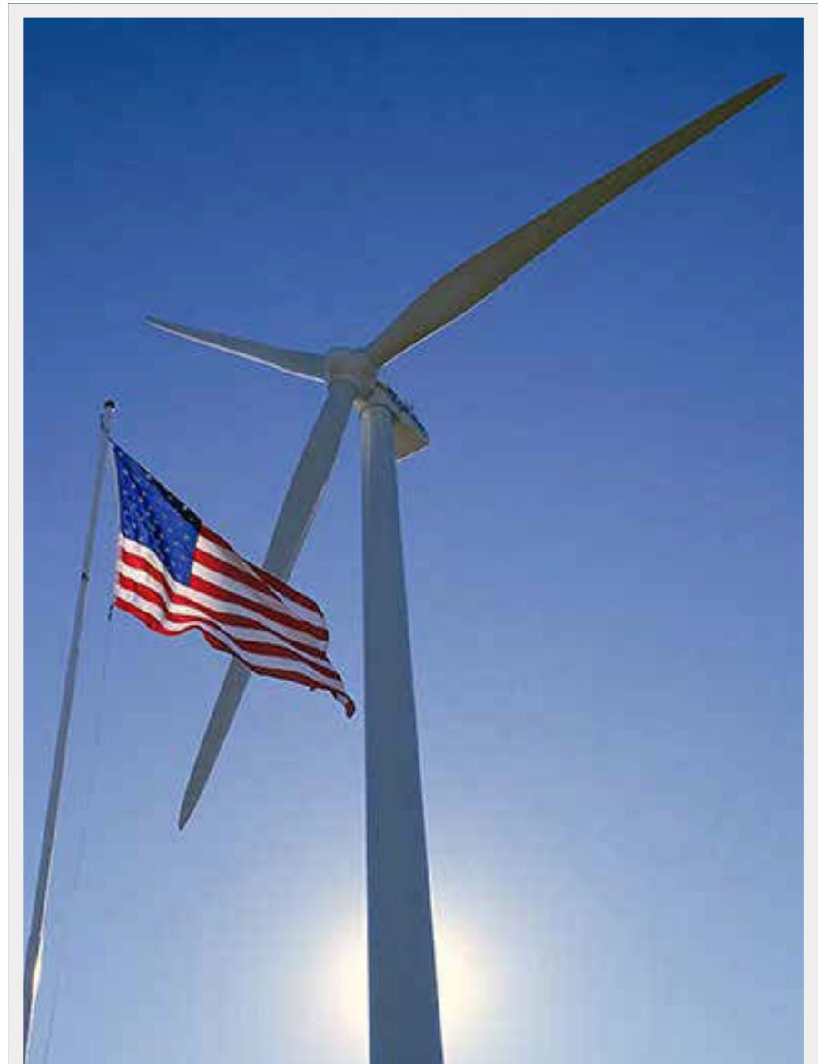
Early coordination with the Federal Aviation Administration, National Oceanic and Atmospheric Administration, Department of Homeland Security, and the U.S. Department of Defense during the siting process can help prevent a radar interference issue long before a wind power plant is built.
