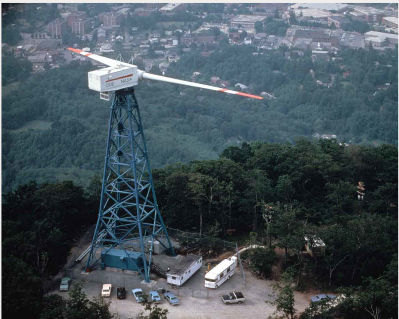
One of the case studies of significant U.S. wind power innovations included in this work focused on a series of test turbines built and operated from 1975 to 1996. Shown here is a 2.2-MW, two-bladed, fixed-speed turbine called Mod-1 but nicknamed "Old Thumper," which in the late 1970s taught lessons on drivetrain reliability, noise, and community engagement. Photo courtesy of the National Aeronautics and Space Administration
