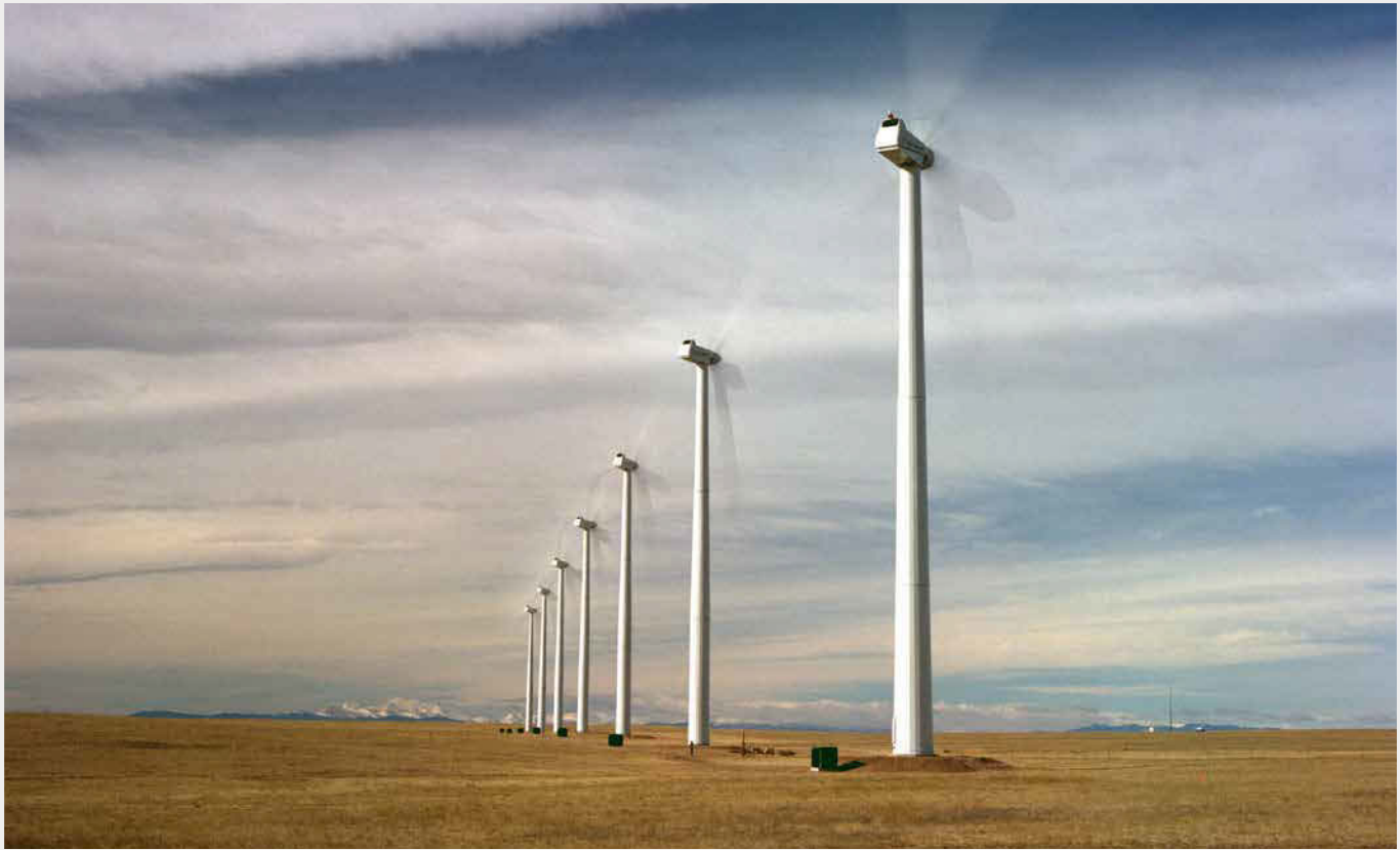
Allowing communication between wind turbines can improve the overall power performance of large-scale wind farms. Photo by Warren Gretz, NREL
