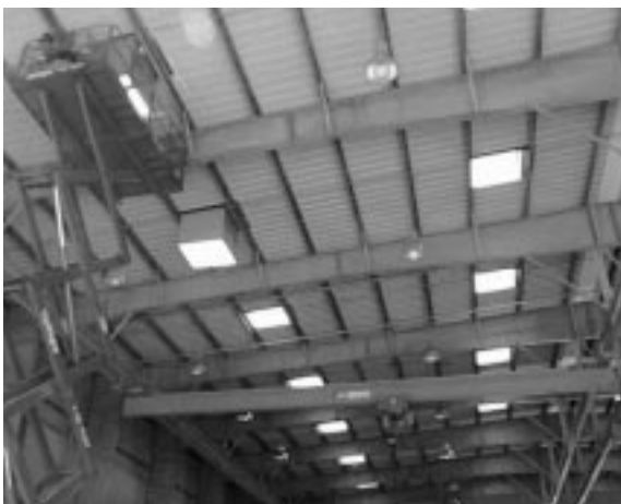
Daylighting retrofits at Wheeler Army Airfield in Hawaii included new skylights for the airplane hangars; skylights like these reduce an agency's electricity bills.
