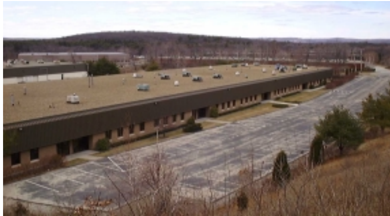
Figure 25 New Factory Building.
