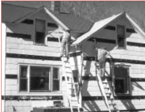
South Dakota crew installs sidewall insulation in a single-family home.
