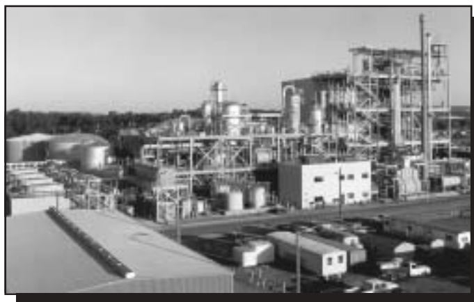
Evergreen Nylon Recycling Plant in Augusta, GA.
