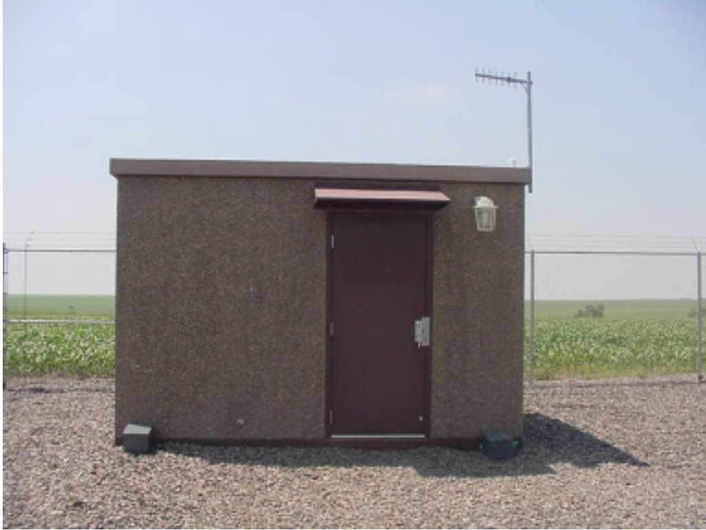
Figure 18. Golf interconnect building
