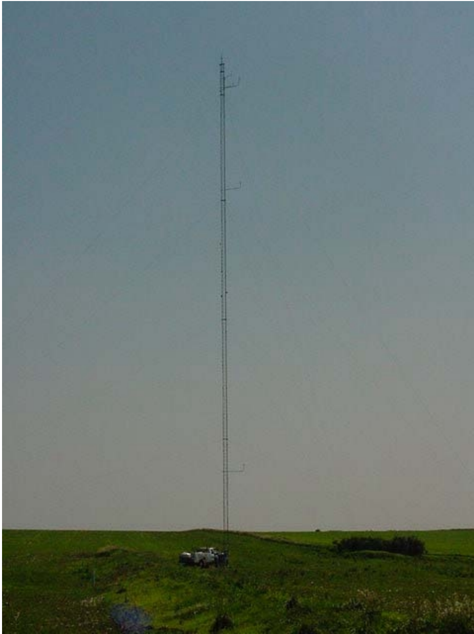
Figure 20. Tower 6 with Met One logger and transducers
