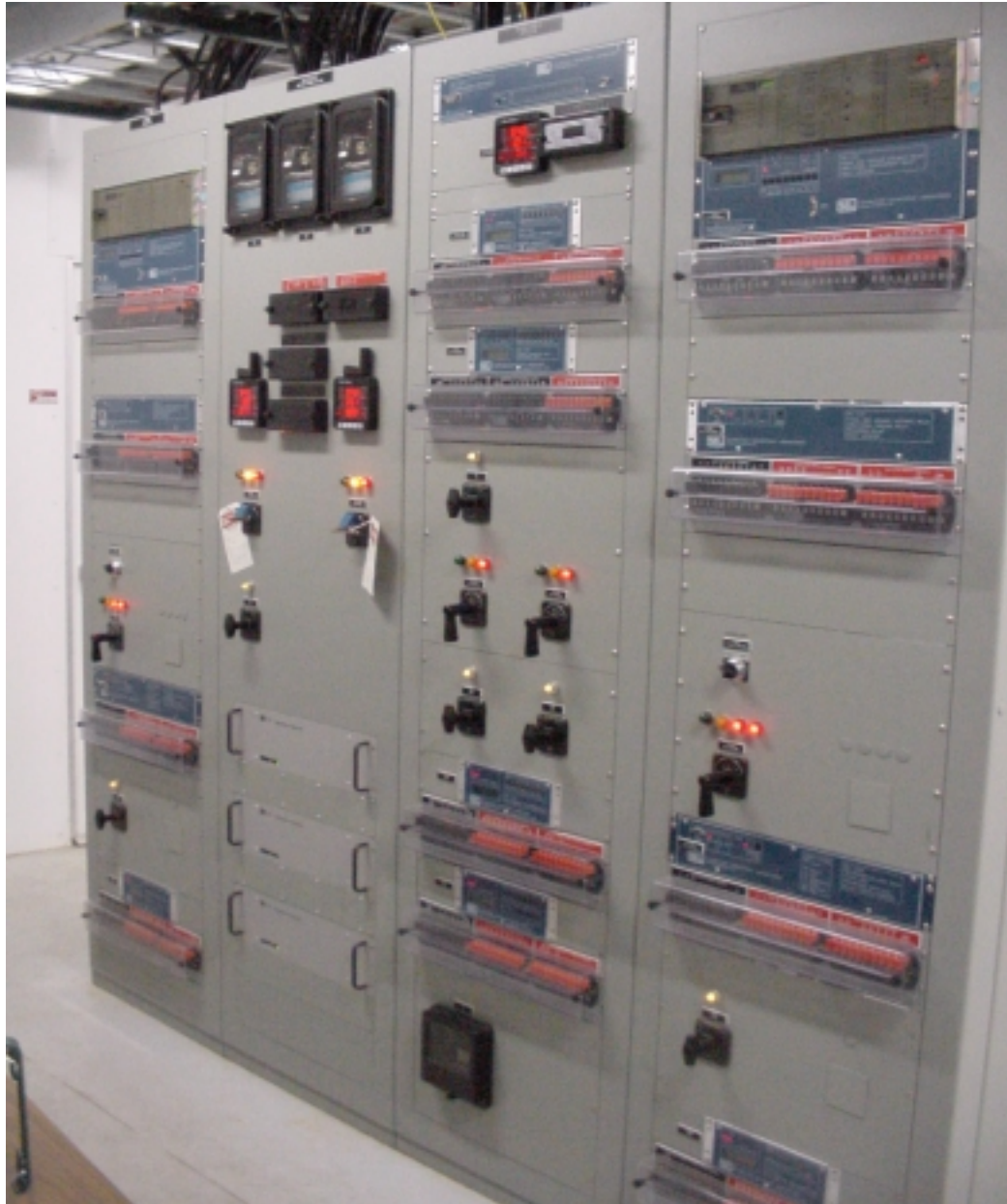
Figure 6. Installation of power monitoring equipment (front)
