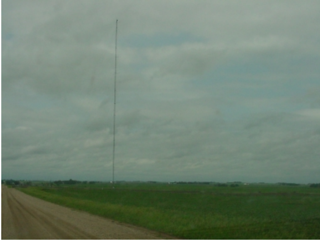
Figure 13. Tower 101 with Met One logger and transducers
