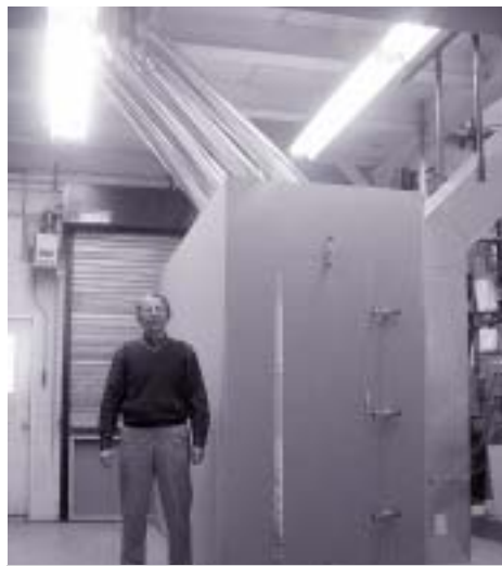
Brookhaven's Residential Duct Laboratory Program Manager John Andrews stands next to the "register box," which simulates the heating load by bringing in cold air from outside. The supply ducts come in from the top and the return duct leaves to the right. The air handler and most of the supply duct system is out of sight on the upper mezzanine level.
