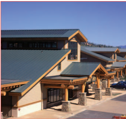
This high-performance commercial building in Silverthorne, Colorado, features roof-integrated photovoltaics, natural ventilation cooling, daylighting, diffusing skylights, and a solar wall—reducing energy use compared to buildings with standard construction. Photovoltaic systems on the rooftops of homes and other buildings are a prime example of how to decentralize power generation.
