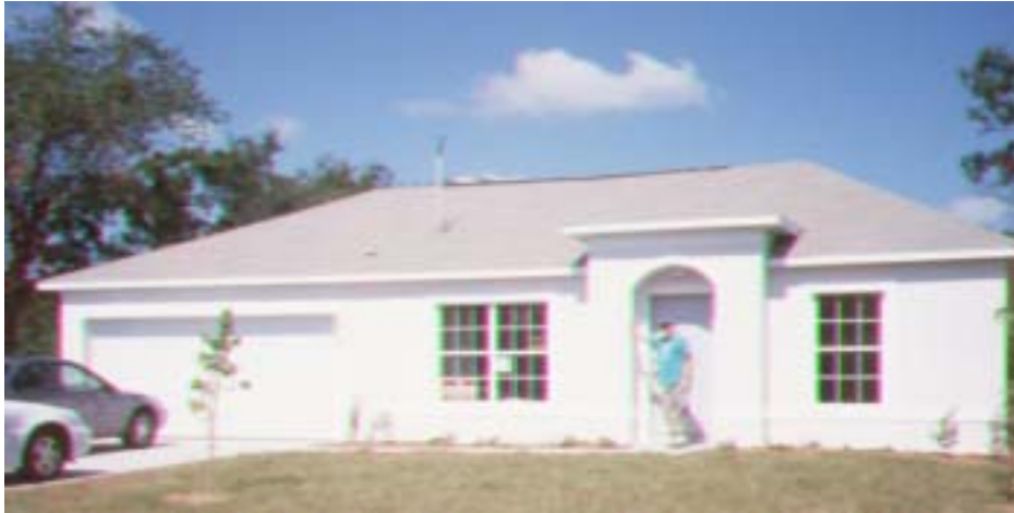
Figure II-9. A Mercedes concrete-wall prototype home
