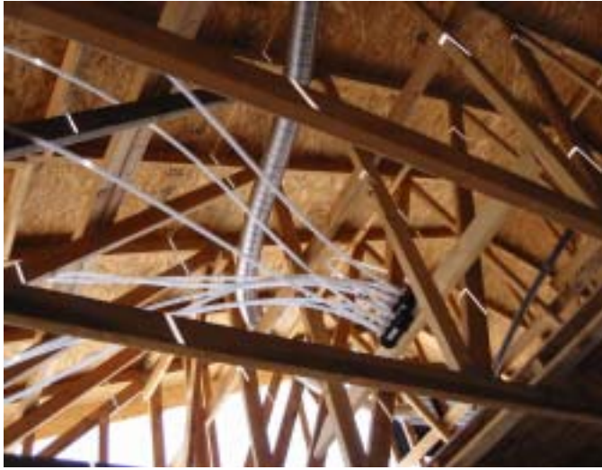
Figure III-13. Domestic hot-water piping (PEX tubing) located in attic and exterior walls
