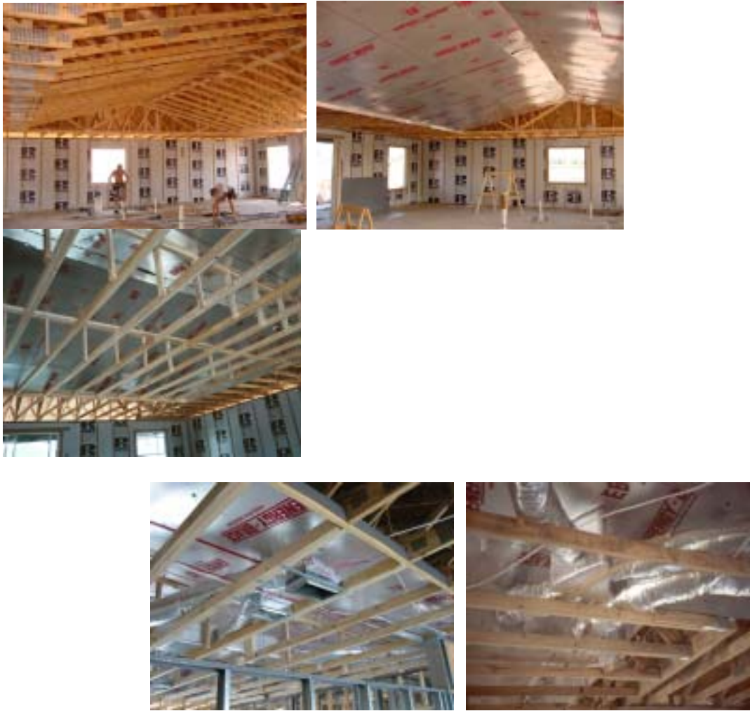
Figure II-31. The revised plenum truss at successive stages of construction
