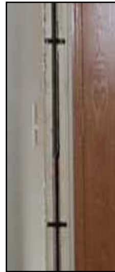
Figure I-44. Gasket seal at marriage wall
