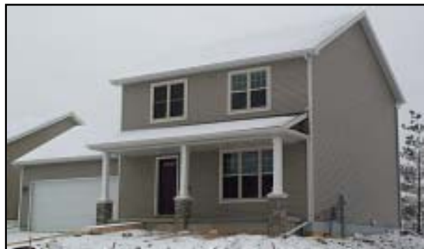
Figure I-21. Newly completed Don Simon Prototype Home
