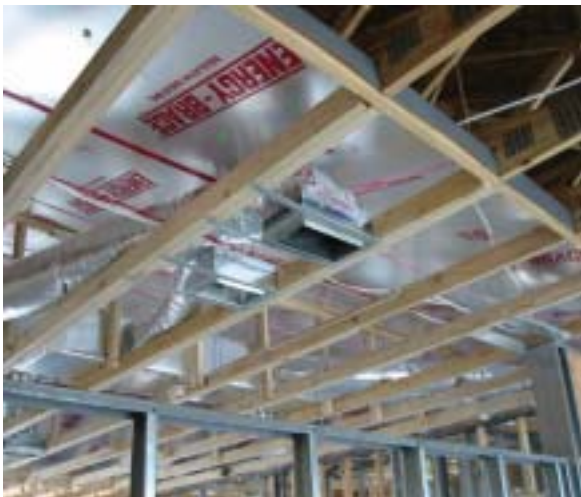
Figure II-5. Plenum truss after lining (left) and after ductwork and lower chord are installed (right)
