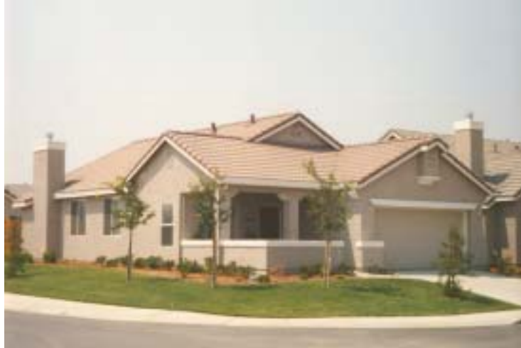
Figure III-1. A CARB house built in a hot-dry climate
