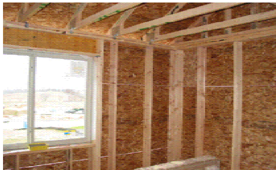
Fig. I-18. In-line framing
