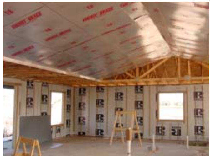
Figure II-5. Plenum truss after lining (left) and after ductwork and lower chord are installed (right)
