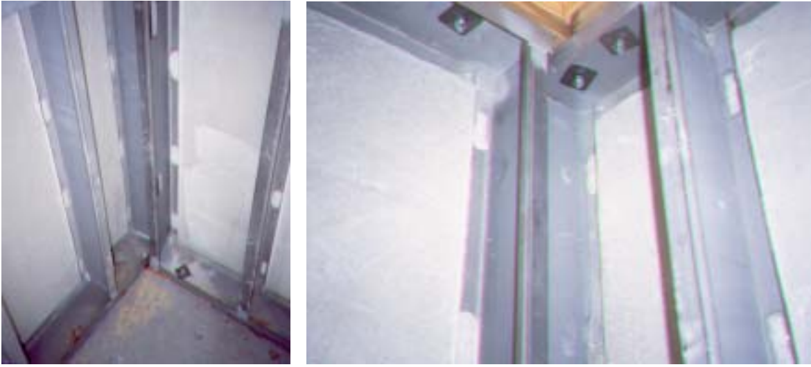
Figure II-11. Ficon panels joining at a corner. Sill is at left, head at right.
