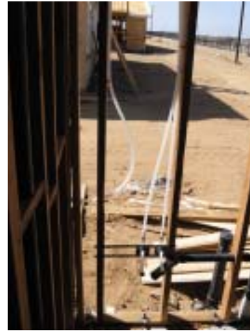
Figure III-13. Domestic hot-water piping (PEX tubing) located in attic and exterior walls
