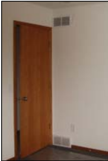
Figure I-24. High and low returns in exterior walls
