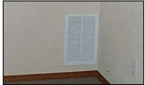
Figure I-36. First-floor low central return
