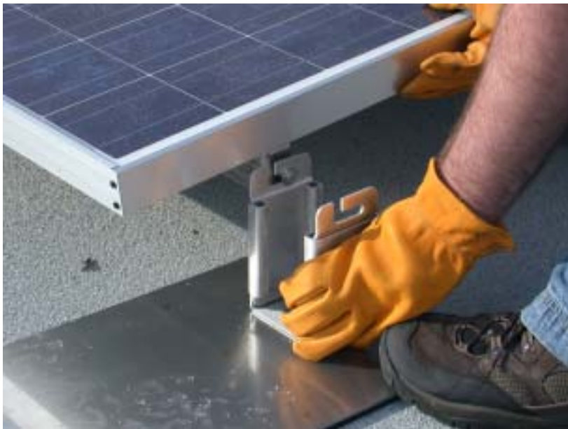
Figure 9. Panel assembly resting in the lower RoofJack.
