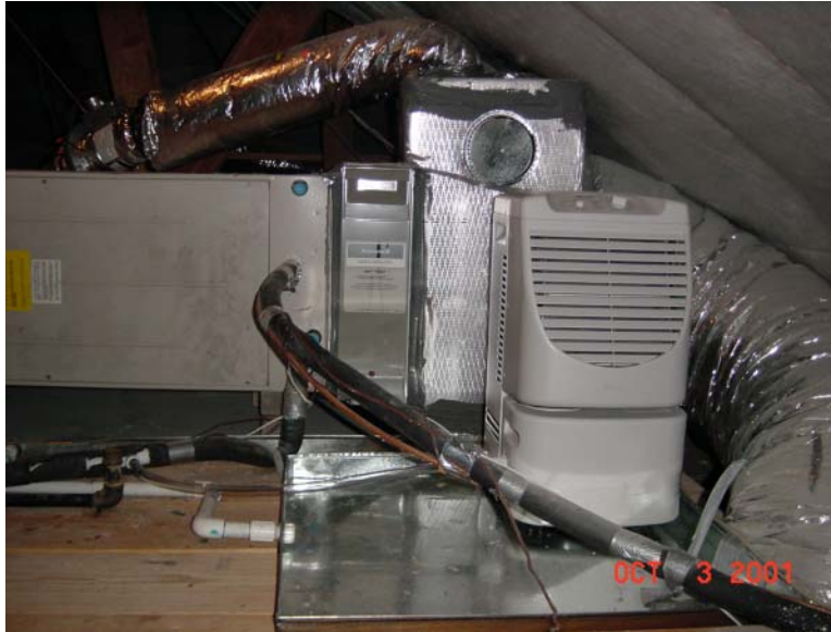
Figure A-2a. Stand-alone dehumidifier in conditioned attic
