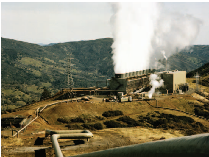
The Geysers in northern California is the world's largest producer of geothermal power. The dry-steam field has successfully produced power since the early 1960s when Pacific Gas & Electric installed the first 11-megawatt plant. The power plant uses NREL's condenser technology to increase operating efficiency. Photo from Pacific Gas & Electric, NREL/PIX 00059
