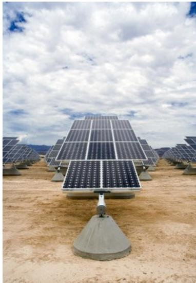
**Figure 2. Ballasted tracking PV system at Nellis Air Force Base, Nevada**
