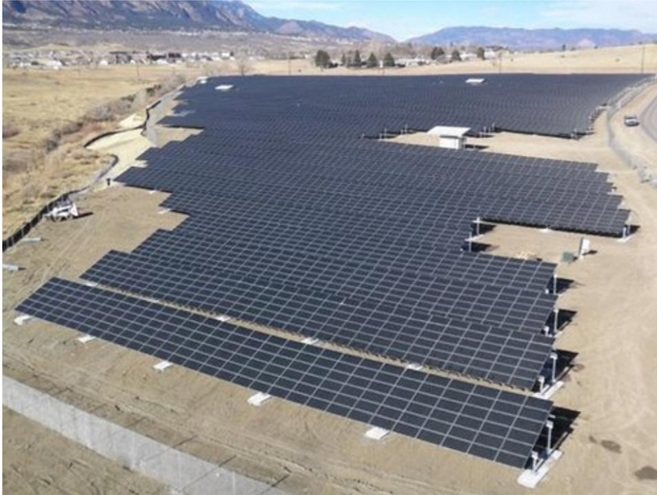
**Figure 1. Aerial view of the 2-MW ground-anchored PV system at U.S. Army Fort Carson, financed through a PPA**
