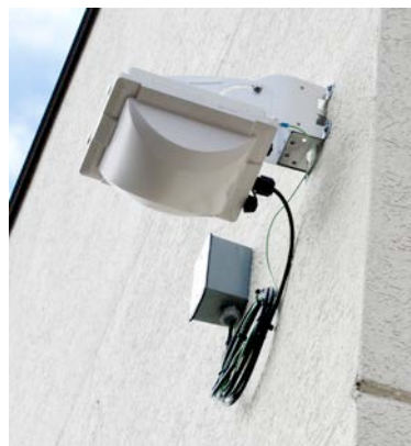
Figure 3. An access point at PPPL. Image Courtesy of PPPL
