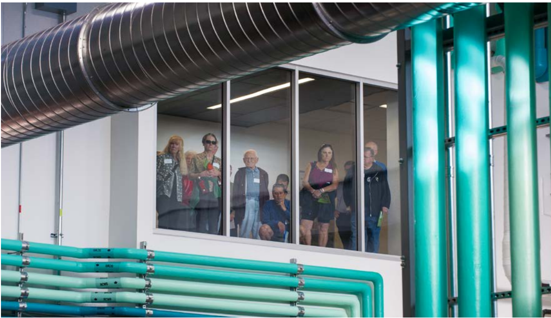
Visitors look into the Power Systems Integration Laboratory during a tour of the ESIF during a Community Open House at NREL.
