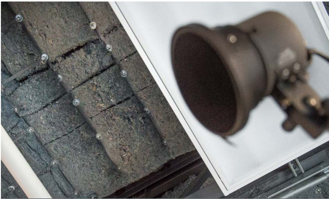
A recycled blue jeans product was purchased to insulate the photo studio on the STM campus as part of the sustainability plan at NREL.
