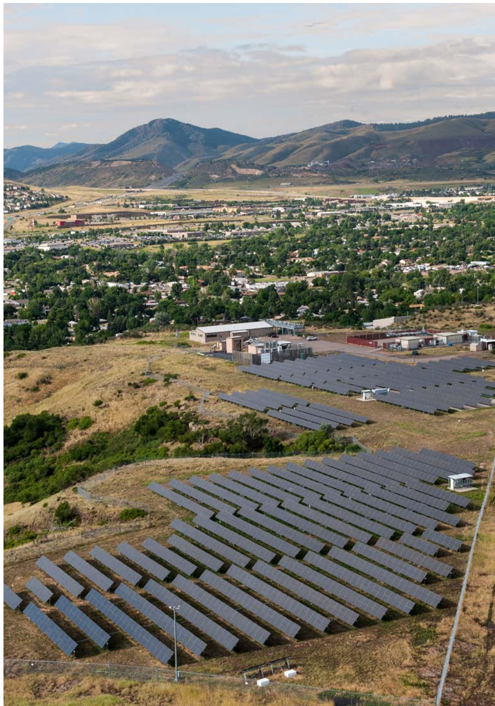
Aerial view of NREL's SRRL and a 720 kW PV array on the mesa top on the STM.
