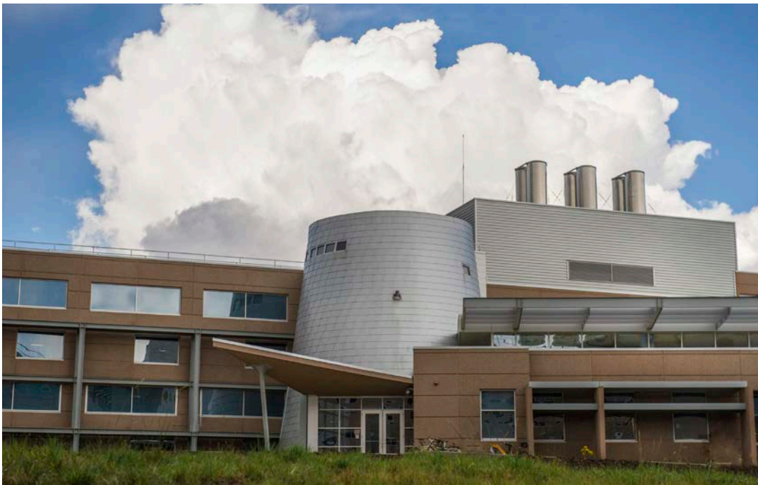
The Science and Technology facility (S&TF) on the NREL campus.
