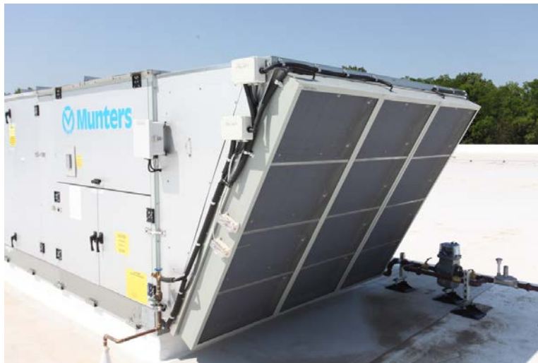
Figure 31. Munters RTU with Evaporcool evaporative condensing installed
