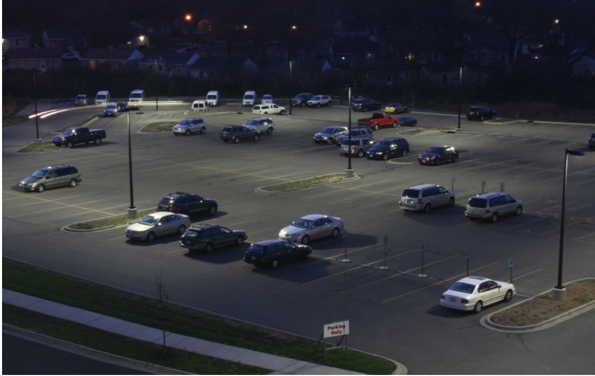
Figure 21. LEDs illuminate surface parking lot in Madison, Wisconsin (Courtesy Rebecca Sadler, Energy Center of Wisconsin)
