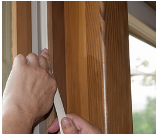
Figure 4. Applying weather stripping to a window
