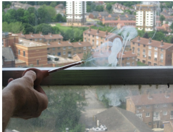
Figure 2. Testing for air leaks with a smoke pencil (Courtesy bob.instituteforsustainability.org.uk)
