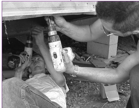
Virginia crew insulates the belly of a mobile home to increase energy efficiency.
