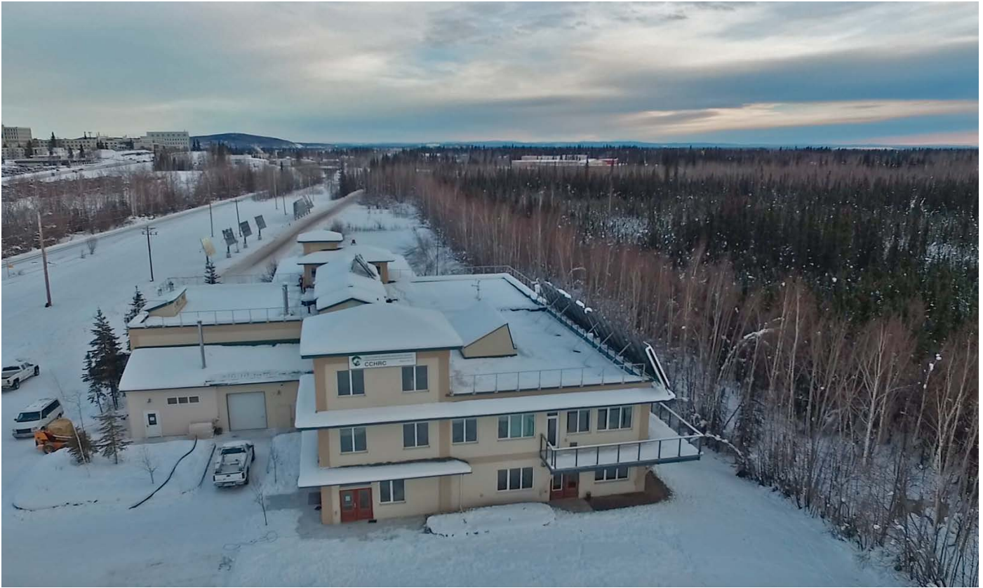
A snowy view of the Cold Climate Housing Research Center in Fairbanks, Alaska. Photo courtesy of the Cold Climate Housing Research Center, NREL 63776
