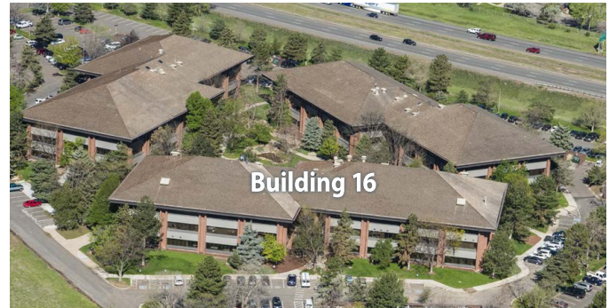
Denver West Office Park, Building 16. Photo by Dennis Schroeder, NREL 44872
