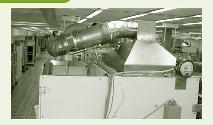
Alzeta's recovery system dramatically reduces the amount of expensive specialty solvents required to manufacture computer disks and other materials by capturing for reuse significant amounts of solvents that would otherwise become greenhouse gas emissions.
