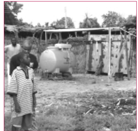
This water purification system for the Nigerian town of Kuje uses a-Si solar panels manufactured by United Solar Systems Corp. to power a UV light disinfection unit manufactured by Waterhealth International, Inc. Capitalizing on the near-Equatorial Africa location, the PV panels are in a flat orientation to capture the sun's direct rays. On each sunny day, the system provides about 1,500 gallons of clean drinking water from a hand-dug well. DOE provided the system in 1999 to promote broad application of similar water-purification systems in Nigeria.
