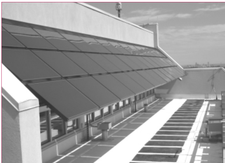
This building-integrated array of 36 amorphous silicon modules from BP Solarex will shade the building and produce 2,250 kWh per year for use in the Outdoor Test Facility at NREL and for delivery to the local utility grid. The system was installed as part of a Cooperative Research and Development Agreement with BP Solarex to study the long-term performance and reliability of the system.
