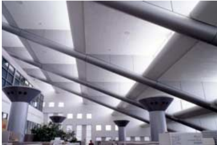
Figure 2. Stepped Clerestory Shelves for High-Quality Daylighting
