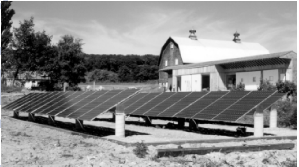
This 11.2-kilowatt photovoltaic array is part of a hybrid solar/diesel generator power system on North Manitou Island, Sleeping Bear Dunes National Lakeshore, Michigan. Three identical subarrays, each with eight strings of nine Siemens Solar M55 PV modules, provide a total peak current of 75 amperes for charging a 288-kilowatt, 120-volt battery bank.
