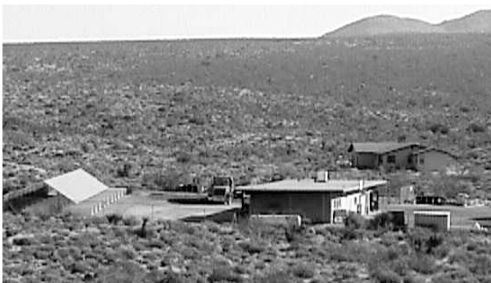
A cost-effective PV array has replaced a diesel system at Joshua Tree National Park's Cottonwood Campground in the California desert.
