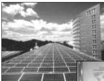
Top photo. BP Solarex high-efficiency panels are powering the headquarters of a leading German financial institution, the Berlin Bank. The panels generate 50 kW peak power and contribute to the bank's energy needs.
