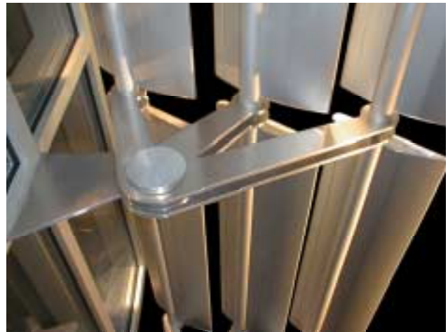
Figure 4. Sunshade structure from underneath.
