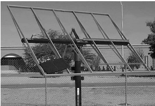
Figure 1: Photograph of a two-axis tracker with no concentrator modules installed
