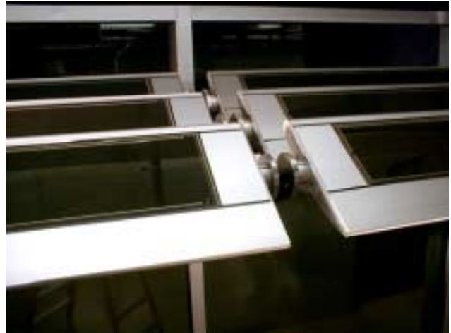
Figure 3. Sunshade blades with thin film modules attached.
