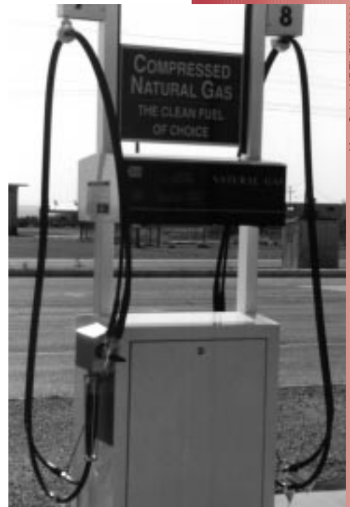
This compressed natural gas station at White Sands Missile Range is one of 14 energy-saving projects under an area-wide contract developed by FEMP in New Mexico that will save the base more than $2 million per year.
