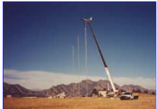
mounting a turbine for testing
