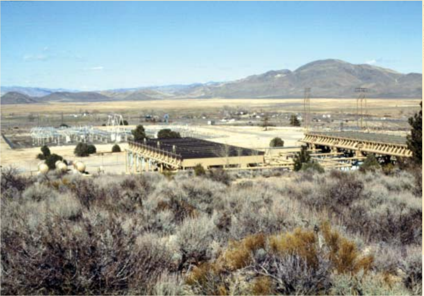
This geothermal plant in Nevada blends well with its environment.
