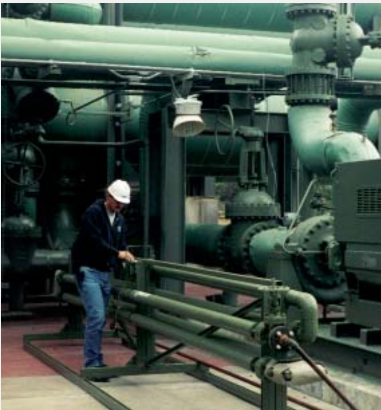
Low-cost polymer coatings are tested in inexpensive carbon steel tubes.
