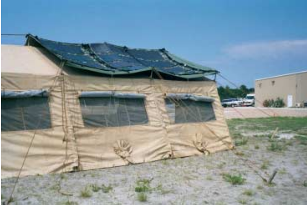
Figure 3. 4 Photograph of TACS Power Storage and Backup Generator System.
