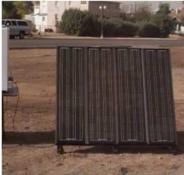
Figure 3. 3 Photograph of a PV array utilizing the GSE Power Flex™ Semi-Flexible Module
