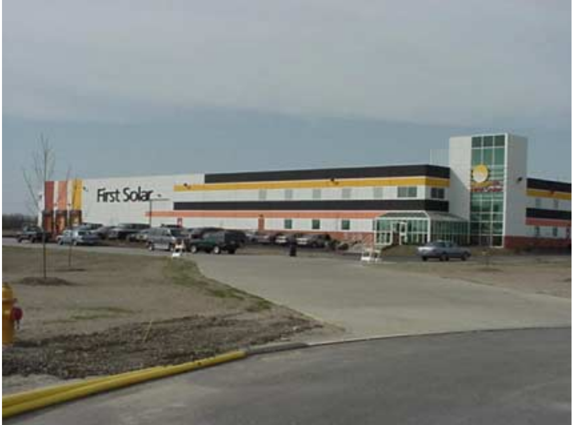
Figure 1. A photograph of the new First Solar 100 MW/year PV module manufacturing plant in Perrysburg, Ohio
