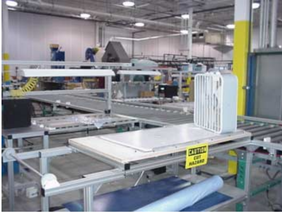
Figure 6. EVA sheet application station before lamination – start of solar finalization line
