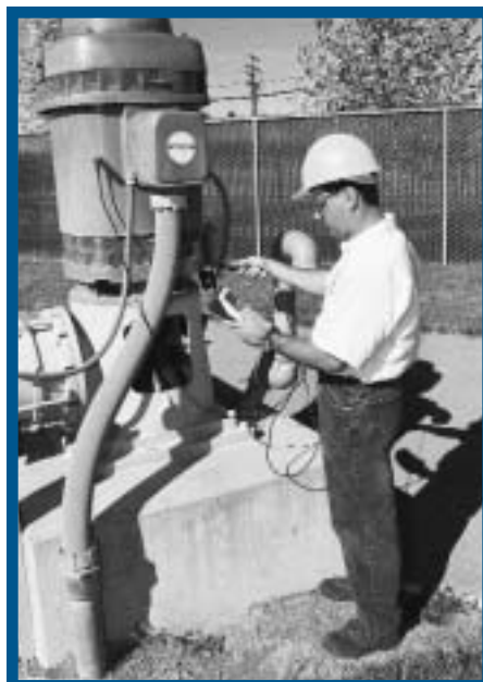
SMUD technical staff tests customers' motors as part of its Motor System Efficiency Initiative.
