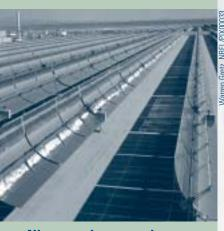
Nine trough power plants in California's Mojave Desert together provide the world's largest solar generating capacity, with a combined output of 354 MW.
