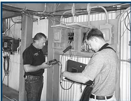
Instantaneous measurements are collected as part of the PAT motor systems analysis.
