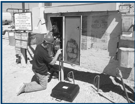
One of the PAT testing team checks connections through the data logger interface.
