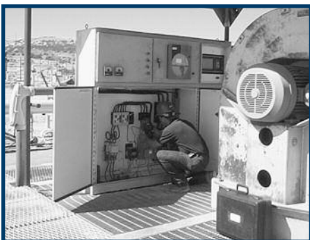
The tester reviews motor data before disconnecting the data logger.
