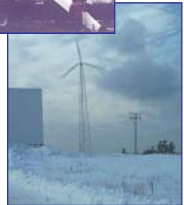
Figure 7. AOC 15/50 wind turbine at the Allen Blueberry Plant in Orland, Maine.
