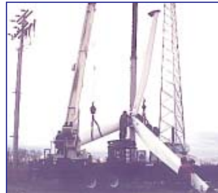
Figure 6. Assembly of the blades into the gearbox.
