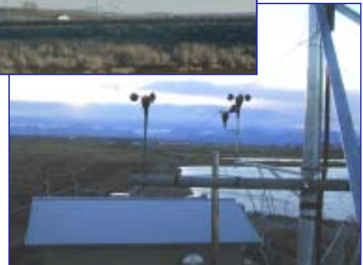
One Bergey wind turbine is on the south side of the aeration ponds next to the pumphouse.
