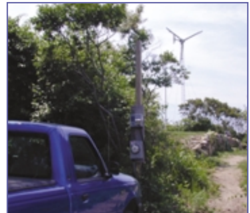
Figure 15. A Bergey 7.5 kW/R wind turbine charges the site's electric Ford Ranger pickup.
