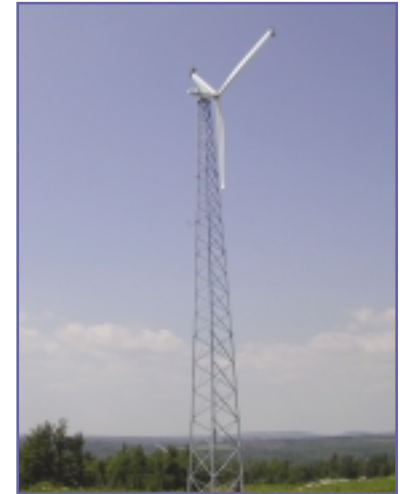
Figure 14. AOC 15/50 wind turbine at the Allen Blueberry Plant in Orland, Maine.
