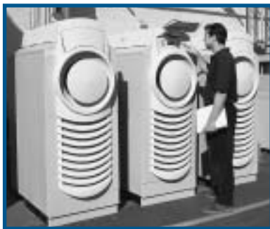
Micro turbines, one example of distributed generation, can be powered by natural gas or biofuels.
