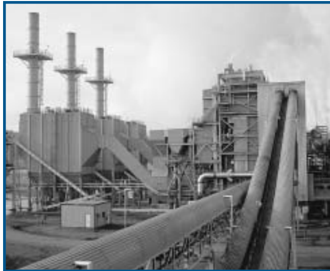
Distributed generation systems, such as biomass generators, can be grid connected or operate independently of the grid.
