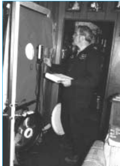
Weatherization workers use the blower door to identify and mitigate air infiltration and pressure imbalances in low-income homes.
