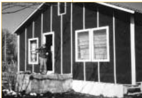
Universal Housing Development Corporation provided extensive weatherization work for this Arkansas home including installing insulation and reducing air infiltration.
