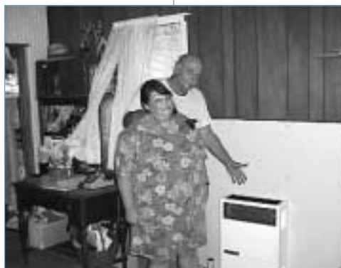
To safeguard this family's health and safety, Weatherization used leveraged funds to install a new heating system.
