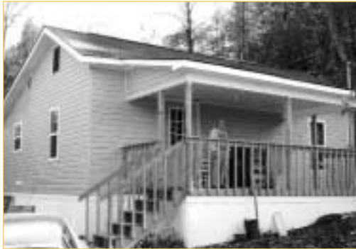
North Carolina provided extensive weatherization services for this home.
