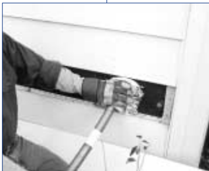
Weatherization crew blows insulation into the walls of a low-income home.
