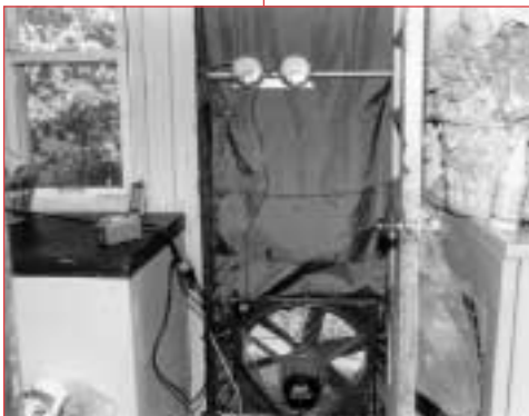
Texas uses the blower door to identify and mitigate air infiltration.
