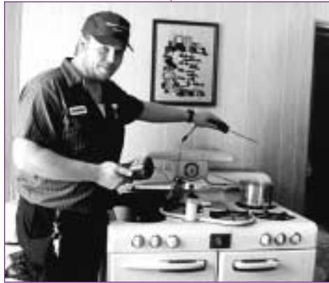
Weatherization technician tests gas range for carbon monoxide.
