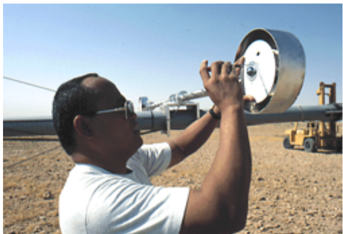
Figure 8.3. Installing IR radiometer in NREL-designed fixture for upwelling IR measurements. Shortwave upwelling radiometer (PSP) on opposite arm.
