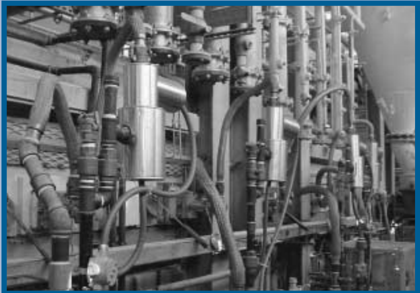
Oscillating combustion technology can produce significant fuel savings, reduce NO x emissions, and can be installed as a simple retrofit, requiring no burner or furnace modification.
