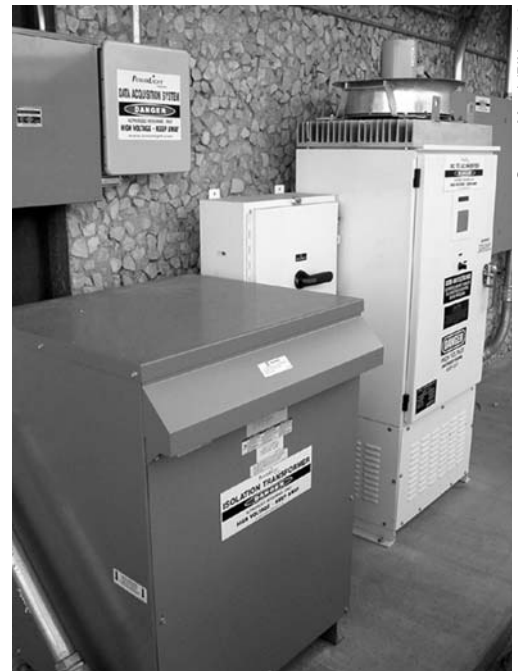
The rooftop solar system at the USPS Marina Center is linked to an energy management system that monitors power output from the PV cells and modifies the building's air-handling and cooling systems, as needed.
