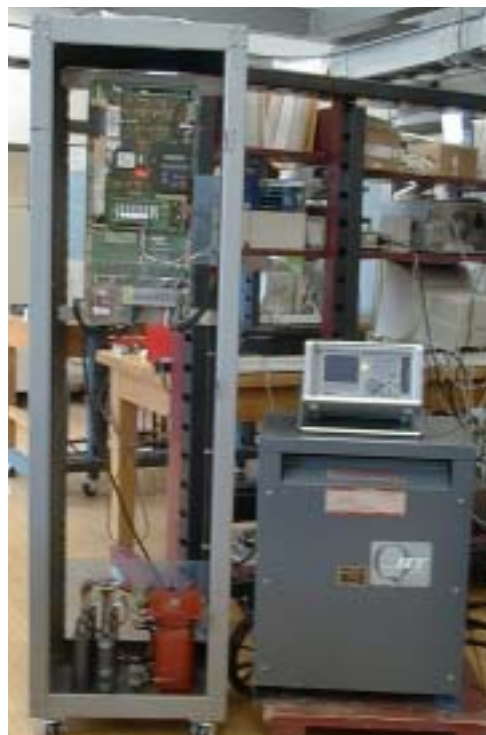
Figure 77: Photograph of inverter incorporating LC filter and transformer
