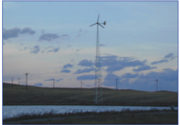
Figure 15. One of the four Bergey Excel 10-kW wind turbines in Browning, Montana.
