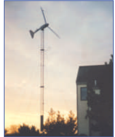
Figure 17. The Bergey Excel 10-kW wind turbine at the Evans Residence, Block Island, Rhode Island.
