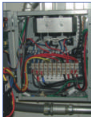
Figure 6. The inside of the EZ Wire.
