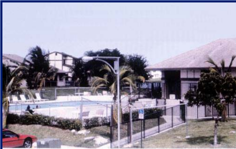
Before Hurricane Andrew, Picture facing N.E.
