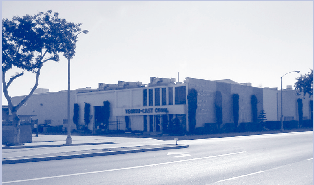
Techni-Cast's plant in Southgate, California
