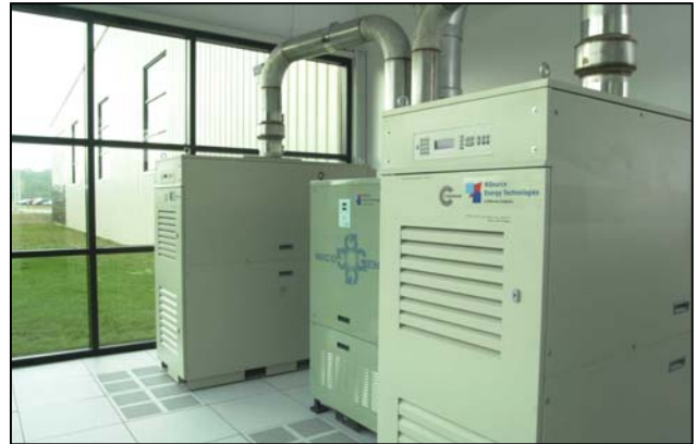
Microturbine CHP installation
